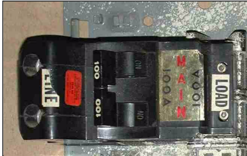
FIGURE 6 - FPE 100-AMP MAIN BREAKER CONNECTS TO THE BUSBARS THROUGH THE PLATE & POST CONFIGURATION, USING ONE SOCKET-HEAD 8-32 SCREW FOR EACH POLE TO ATTACH TO ITS CONTACT PLATE.
